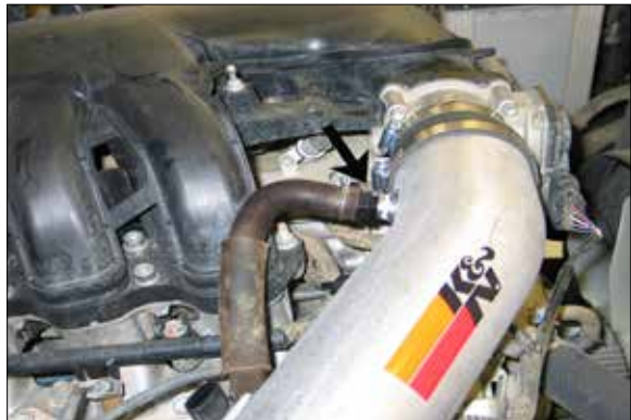
27. Connect the crank case vent line to the 5/8 vent fitting and secure with the factory spring clamp.
